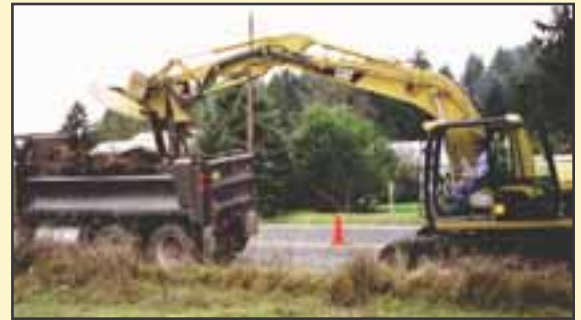
Loading debris for disposal with integrated material handler
